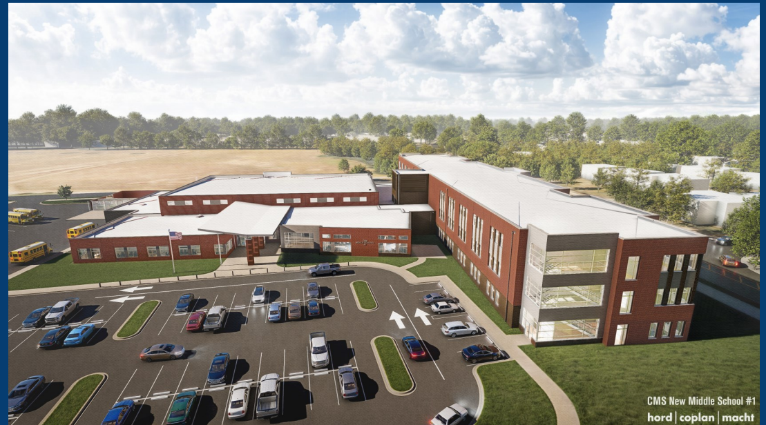
New Middle School 1 South
